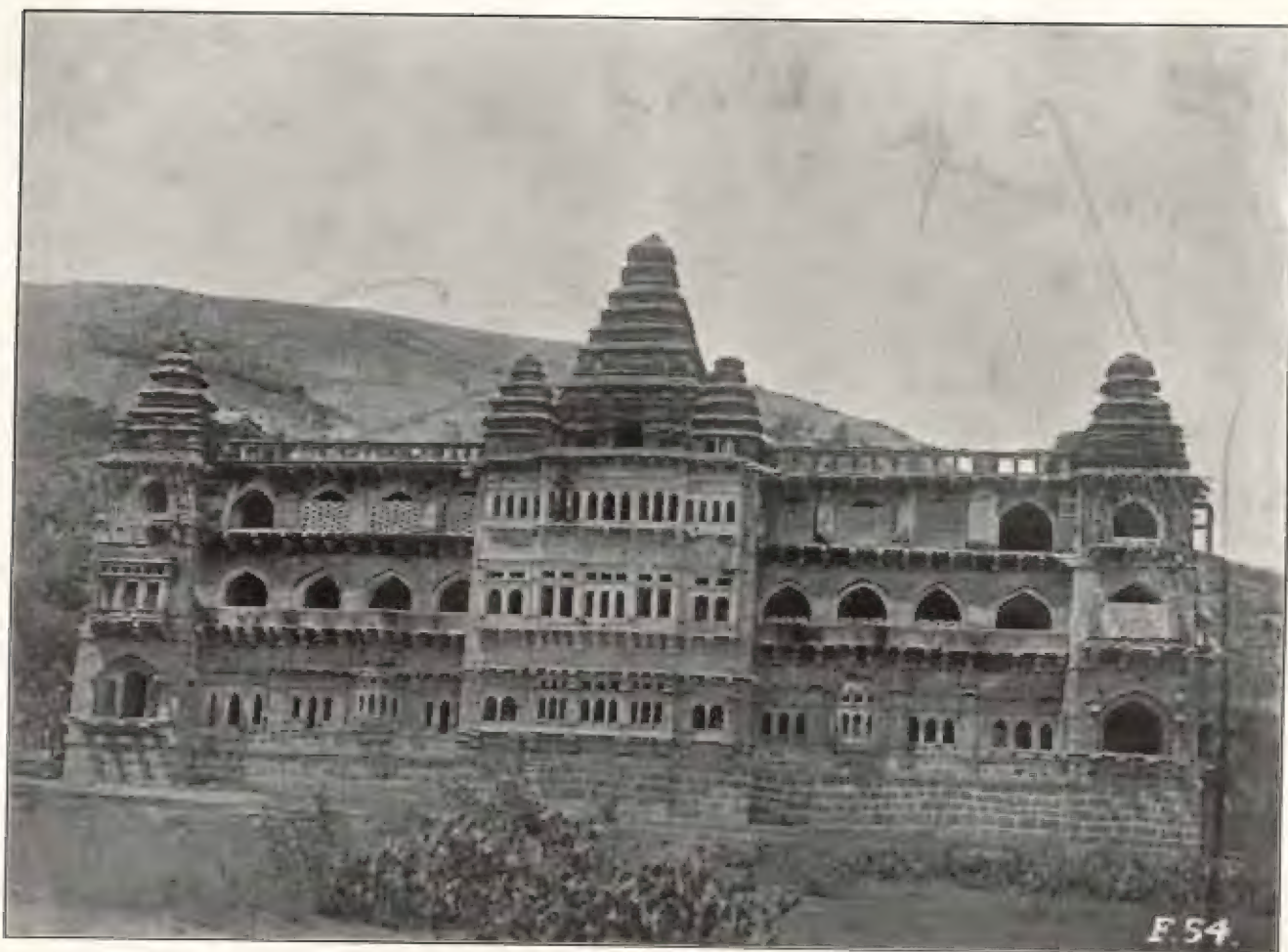
a. KING'S PALACE, SOUTH ELEVATION, CHANDRAGIRI, CHITTOOR.
